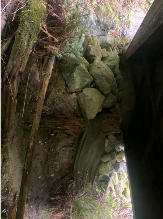
Left Bank Abutment when facing downstream
